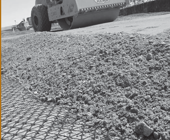
Image 10 Compacting the aggregate fill.
