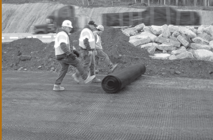
Image 2 Rolling out Tensar® TriAx® Geogrid.
