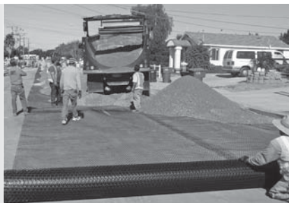
Image 3 Tensar TriAx Geogrid should overlap in the direction of advancing fill.
