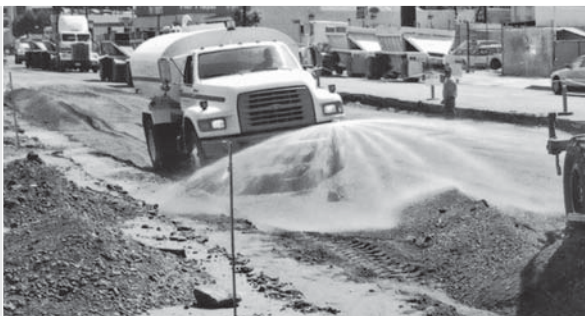
Image 9 Moistening the fill before compaction.
