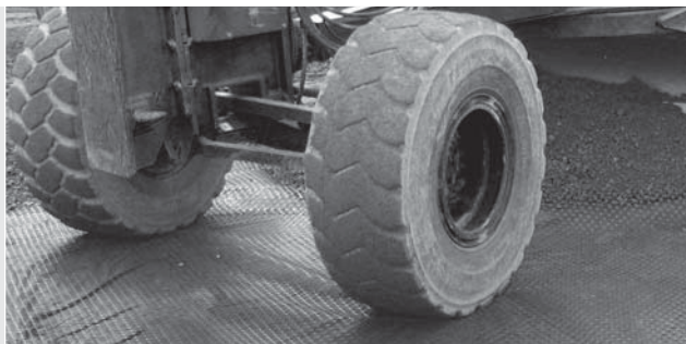
Image 11 Tensar TriAx Geogrid can be trafficked directly by rubber-tired equipment.
