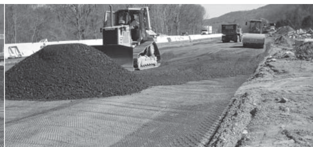
Image 8 Spreading aggregate fill over Tensar TriAx Geogrid.
