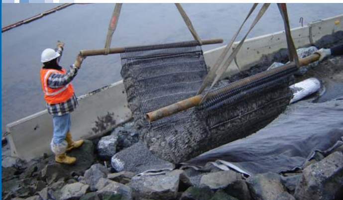
The Triton Mattresses protect the underlying CETCO® Reactive Core Mat®
