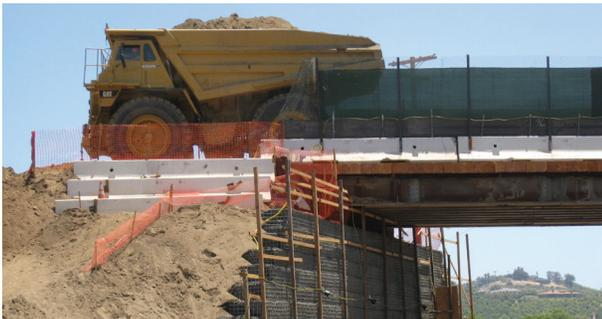
A CAT 777 weighing approximately 360,000 lbs is supported by a Tensar Temporary Wall as it drives to the embankment site.
