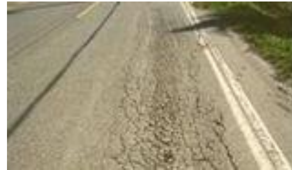
Extreme fatigue cracking/unstable base
