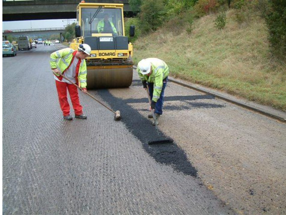
Filling excessive voids after milling the surface
