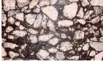
PCC Joint Cracking
