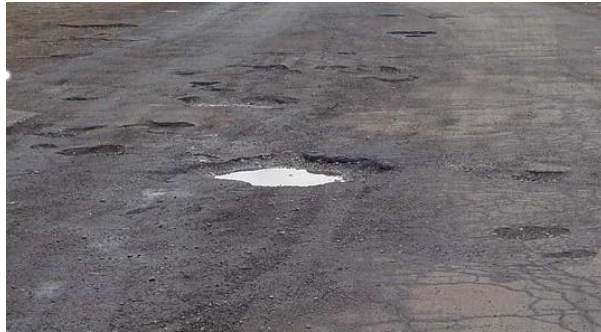
Base Failures
