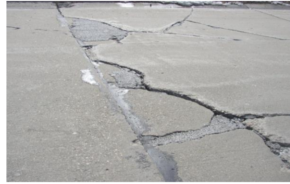
Slab Fracture/Uneven
