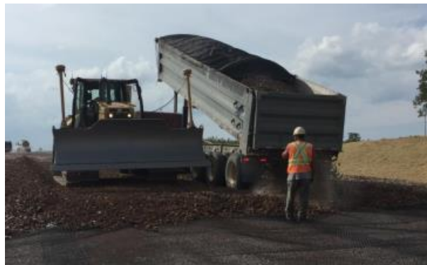
Figure 1. Placement of the aggregate on the geogrid
