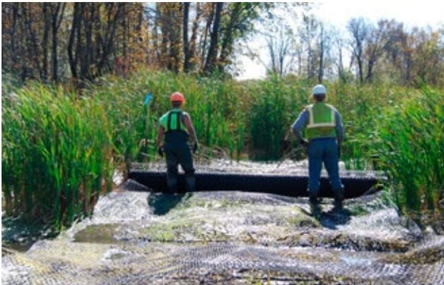
*A layer of Tensar® TriAx® Geogrid was placed directly at the base of the berm to bridge the lake sediment.*
