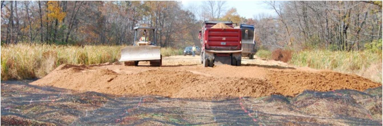
*TriAx Geogrid created an unyielding and stable platform for constructing the berm.*
