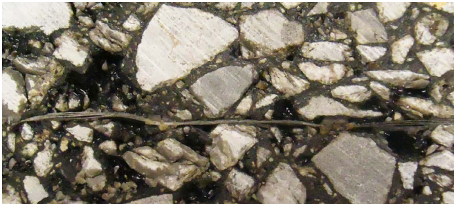
Core sample showing GlasGrid 8501 bonded to the sandwiching layers of SMA mix.
