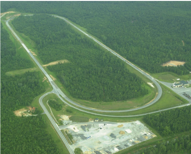
The GlasGrid Pavement Reinforcement System was installed at the National Center for Asphalt Technology (NCAT) pavement test track in Opelika, AL.
