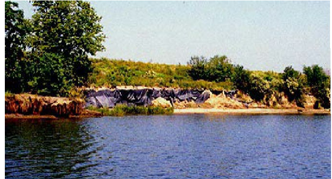
Fig. 1: Bluff eroding into containment dike along north bank immediately upstream from test sites. Geotextile was previously placed within embankment.
