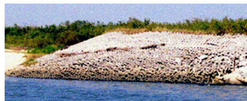
Figure 15: Washout of tetrapod units at downstream flanking of Section E. Failure appears to have developed from the toe.
