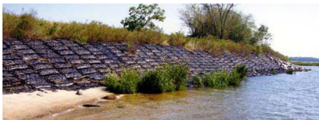
Fig. 18: Marine Mattress Section F looking downstream. Stability has been maintained throughout.
