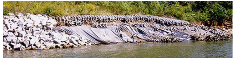
Figure 15: Washout of tetrapod units at downstream flanking of Section E. Failure appears to have developed from the toe.
