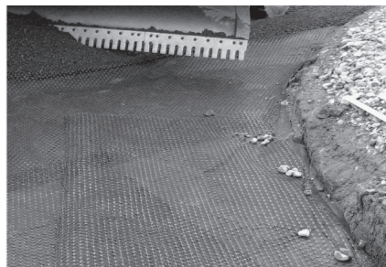
Placing Geogrid to accommodate curves.
