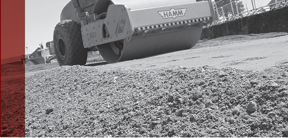
Compacting the aggregate fill.
