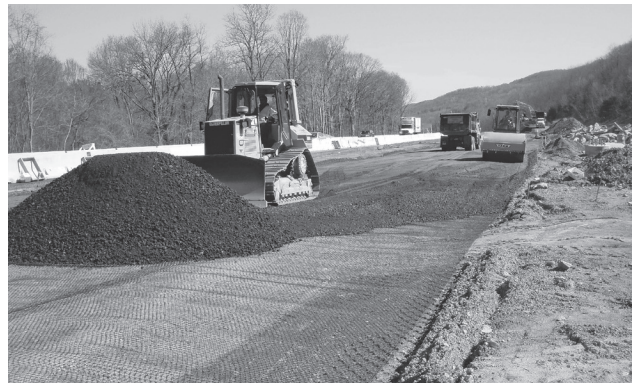
Spreading aggregate fill over Tensor Geogrid.
