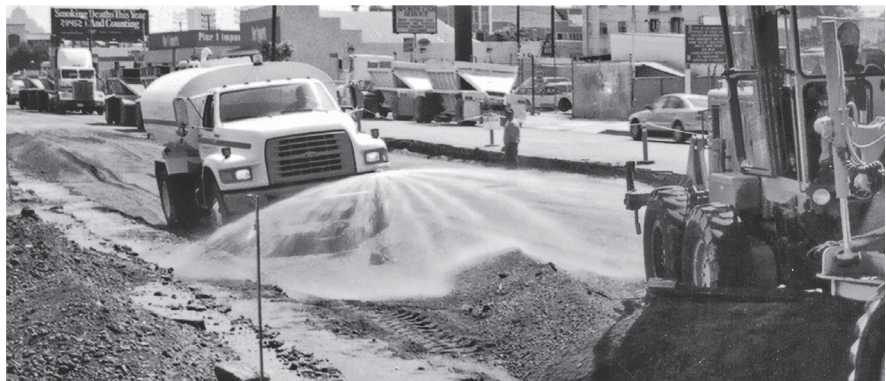
Moistening the fill before compaction.
