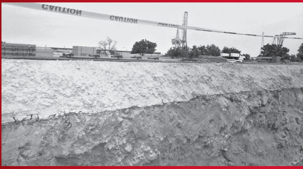
A backhoe excavation through Tensar Geogrid.
