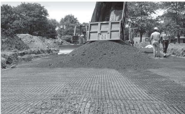
End dumping aggregate fill on top of Tensor Geogrid over soft subgrade.
