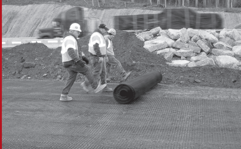
Rolling out Tensar® Geogrid.
