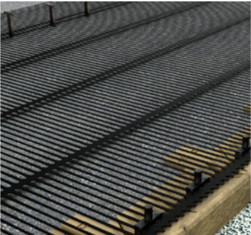
Once the connectors and the geogrid are in place, the Olympia® Units must be swept clean prior to placing the next course. Failure to do this can result in problems with seating and leveling of subsequent courses.
