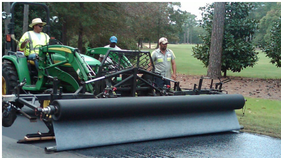
Image 1: Interlayer laydown equipment.
