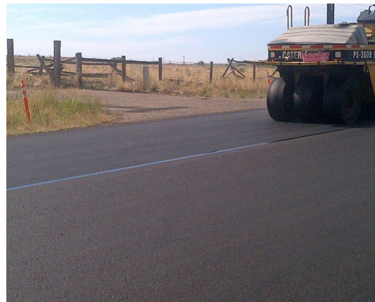
Image 4: A pneumatic tire roller is recommended to bond the GlasPave mat to the tack coat in certain scenarios.
