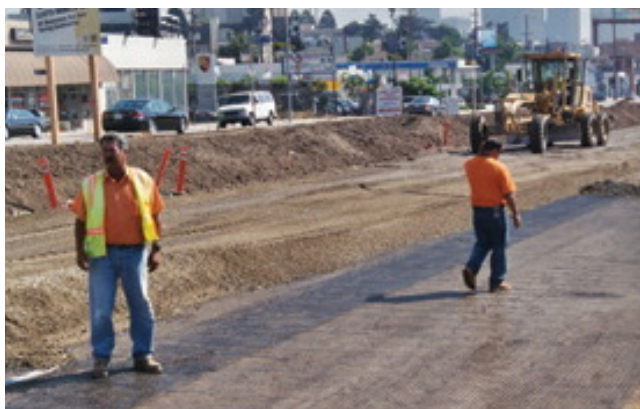
Geogrid-reinforced sections of Palomar St. and Industrial Blvd., two high-volume roadways in Chula Vista, outperformed comparable unreinforced sections over a five-year period.
