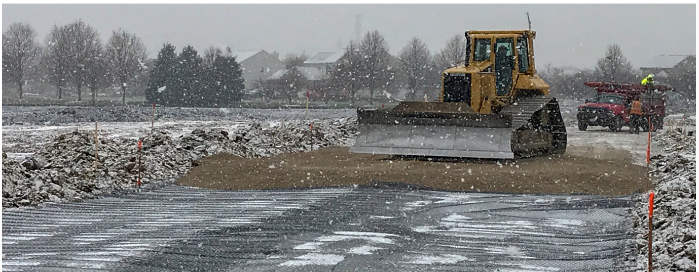
In the Northpointe Subdivision project, the contractor encountered soft soils during excavation. Due to cold weather, the Village of Plainfield, IL does not allow lime stabilization after October 15th. A TX5 geogrid solution required no undercut to stabilize the subgrade and allowed construction to continue through cold weather conditions.
