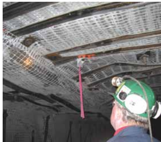
NIOSH tested Tensor UX3326-45 Geogrid against 8-gauge, welded wire mesh.
