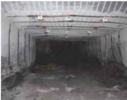
The easy-to-install, white, reflective Tensor® Roof Mat is corrosion-resistant and flame retardant.
