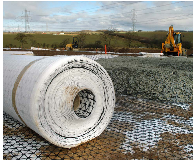
The high profile ribs and nodes of TriAx geogrid allow full aggregate strikethrough when combined with a nonwoven geotextile..
