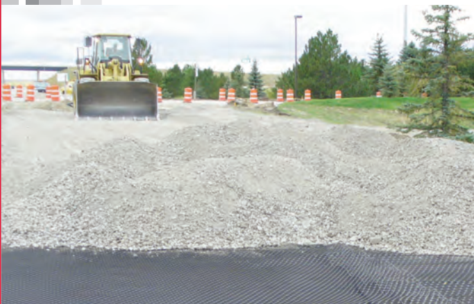
Tensar ® TriAx ® Geogrid enabled a major reduction in the volume of imported granular fill.
