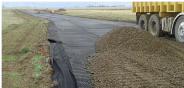
Installation of Tensar TriAx160 reduced aggregate requirements of access roads
