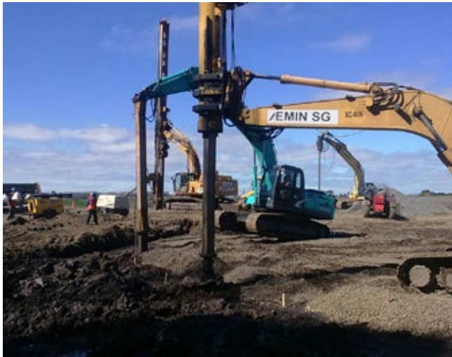
Installation of Geopier Rammed Aggregate Pier Elements
