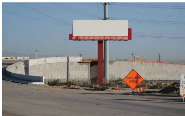
Carretera Eastgate – Henderson, Nevada
