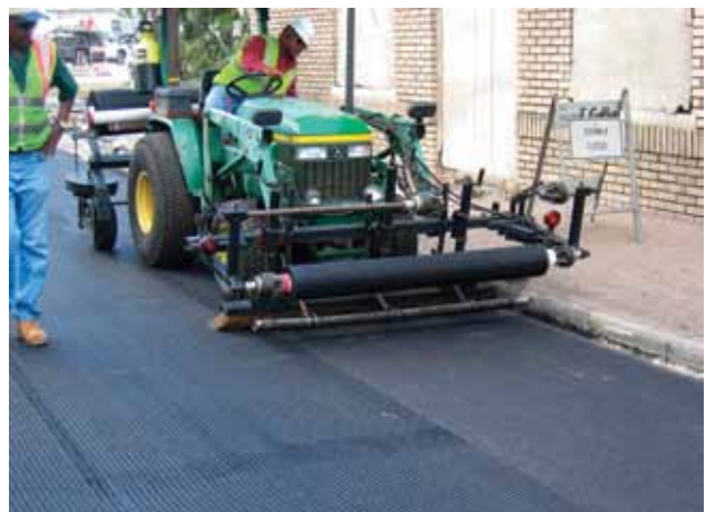
A GlasGrid full width installation using a high speed, 5 ft wide installation device.
