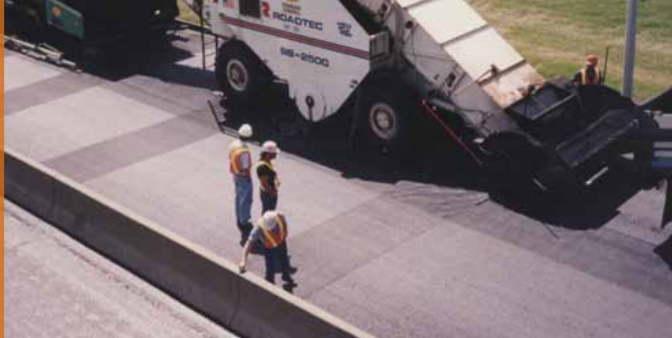
GlasGrid detail repair installation where an asphalt transfer device is used as part of the paving train.
