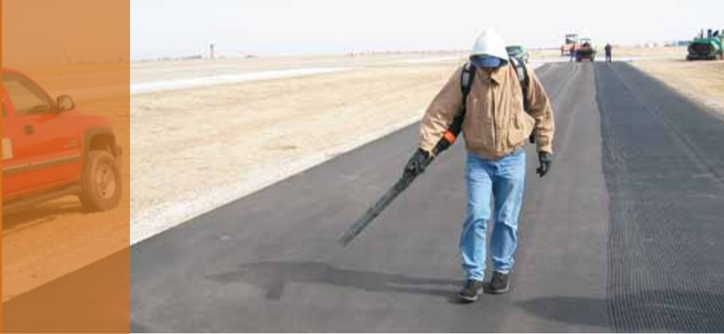
Surface preparation includes blowing off any dust before installing the self-adhesive GlasGrid System.
