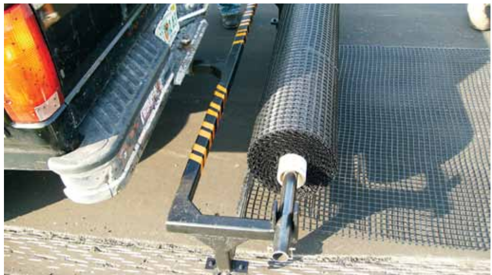
IMAGE J: GlasGrid rolls can be installed manually for smaller pavement areas.
