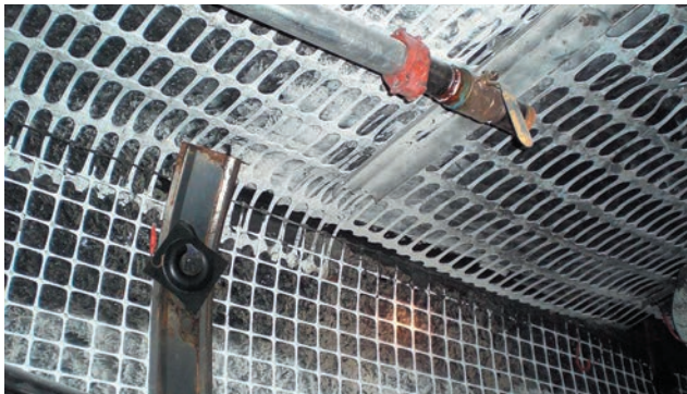
Tensar® BX and UX Mining Geogrids provide effective roof and rib control for soft minerals as well as the most demanding hard rock and tunneling applications.
