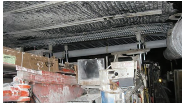
Tensar® TriAx® Geogrid can be installed without brackets, thus eliminating unnecessary downtime.
