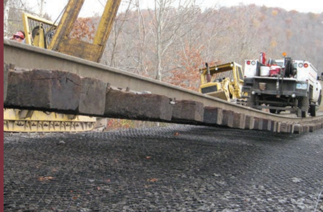
IMAGE D: Existing track can be jacked up so that new geogrid and ballast can be added.
