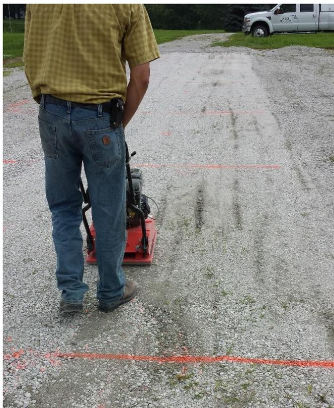
**Figure 7. Vibratory compaction of aggregate base layer prior to APLT for uniform and level testing surface.**
