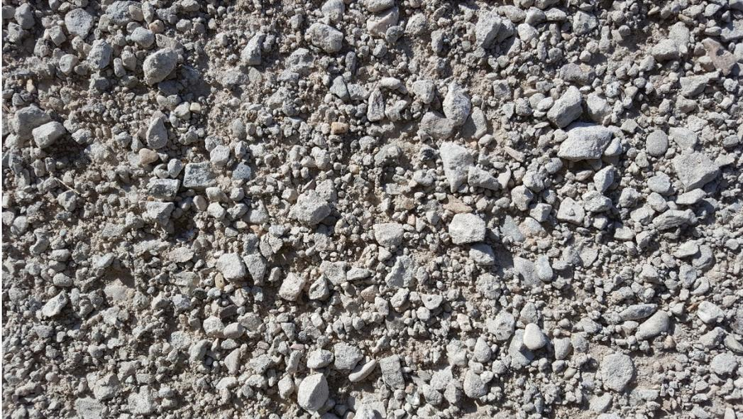
**Figure 9. Compacted recycled concrete aggregate (RCA) over TX160 geogrid (May 9, 2016).**
