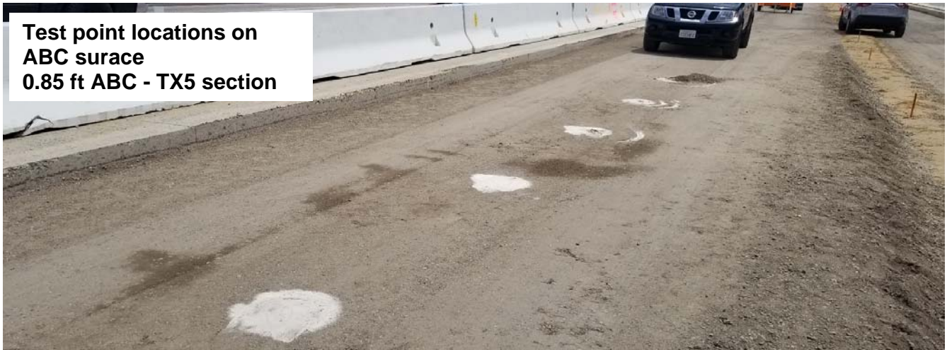
TX5 Geogrid at the base/subgrade interace 0.85 ft ABC - TX5 section
