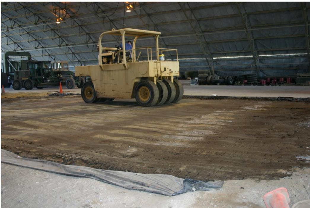
The crushed limestone material was placed in 8- to 10-in. lifts and compacted using a large vibratory steel-wheel roller. Figure 4 shows the crushed limestone material being dumped in place, while Figure 5 shows the material being compacted.
