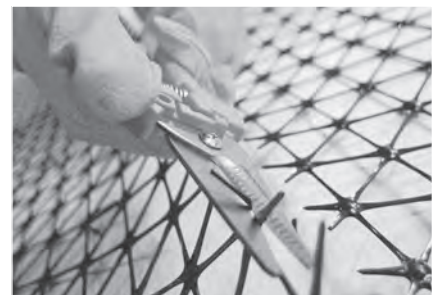
IMAGE 5: Cutting Tensor TriAx Geogrid is easily achieved.
