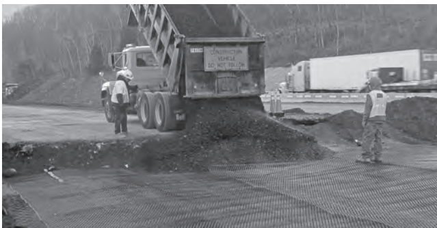
IMAGE 7: End dumping aggregate fill on top of Tensar TriAx Geogrid over soft subgrade.
