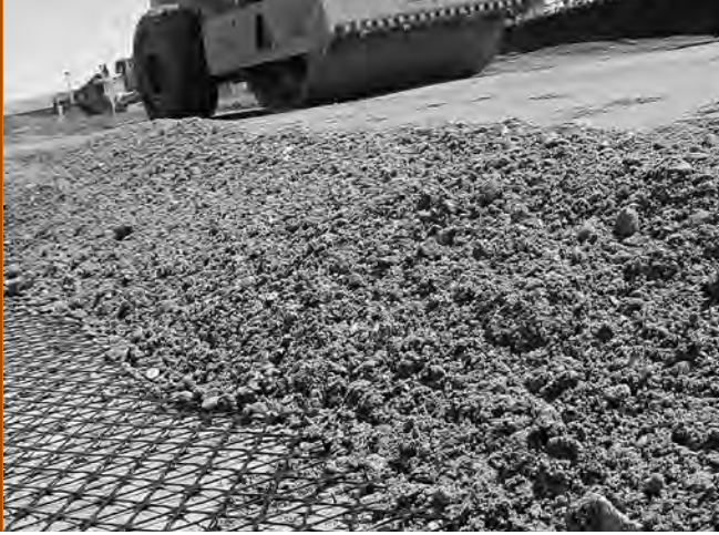
IMAGE 10: Compacting the aggregate fill.
