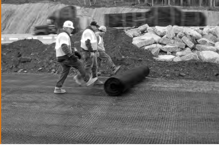
IMAGE 2: Rolling out Tensor® TriAx® Geogrid.
