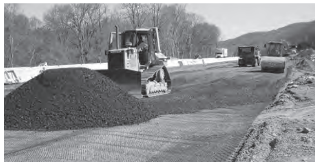
IMAGE 8: Spreading aggregate fill over Tensar TriAx Geogrid.
