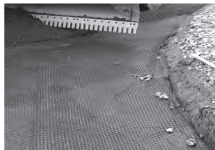
IMAGE 4: Placing Tensor TriAx Geogrid to accommodate curves.
