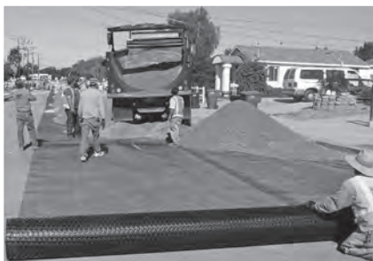
IMAGE 3: Tensor TriAx Geogrid should overlap in the direction of advancing fill.
