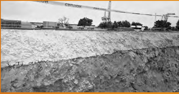
IMAGE 12: A backhoe excavation through a Tensar TriAx Geogrid.
