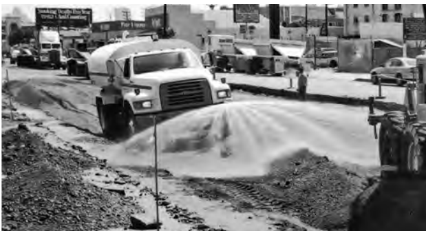
IMAGE 9: Moistening the fill before compaction.
