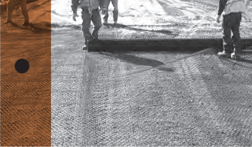
Overlapping Tensor® TriAx® Geogrid in the field is quick and easy.
