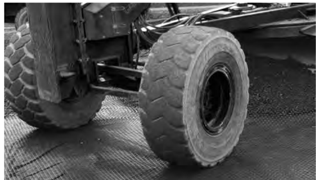
IMAGE 11: Tensar TriAx Geogrid can be trafficked directly by rubber-tired equipment.
