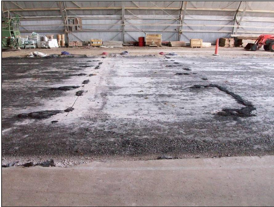
Photo 2. Asphalt strain gauges were covered with cold patch prior to paving operations
