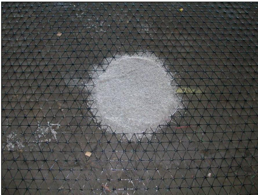
Photo 4. Gauges were covered with sand to prevent damage during base course installation.
