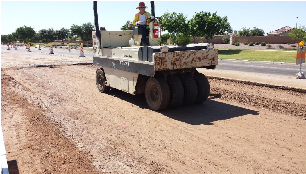
Figure 9. Pneumatic tired roller used just prior to testing (April 17, 2015).
