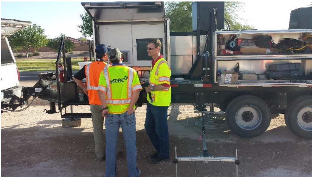
Figure 10. APLT testing at 30 in. static test point (April 17, 2015).
