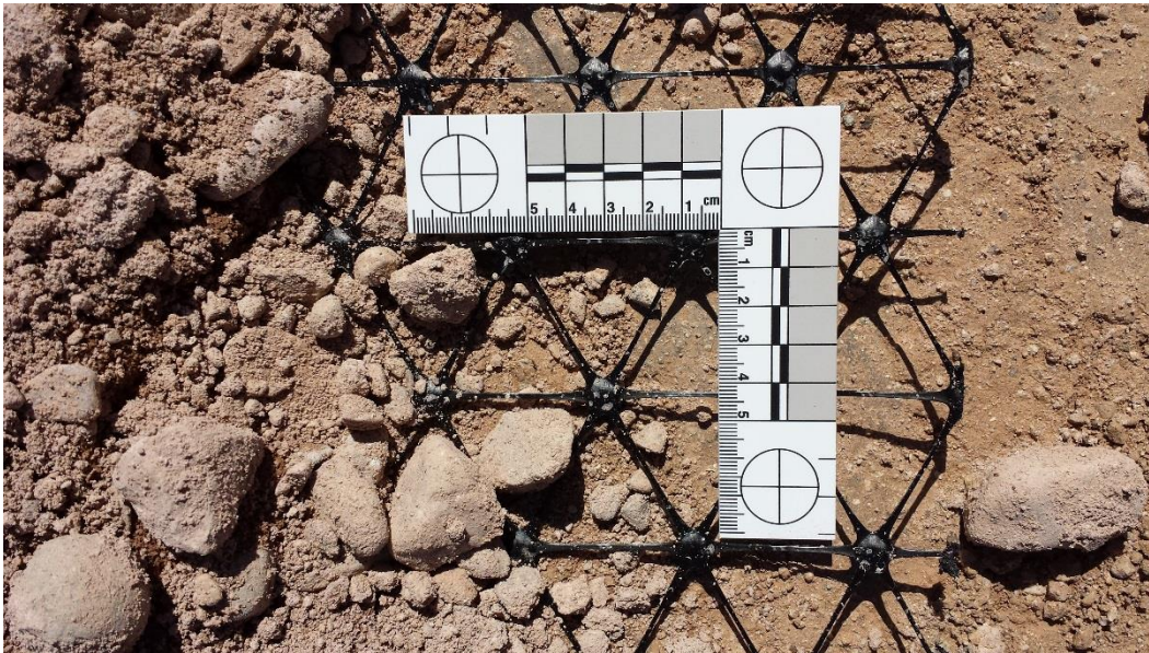
Figure 8. Aggregate base course over TX5 (April 17, 2015).
