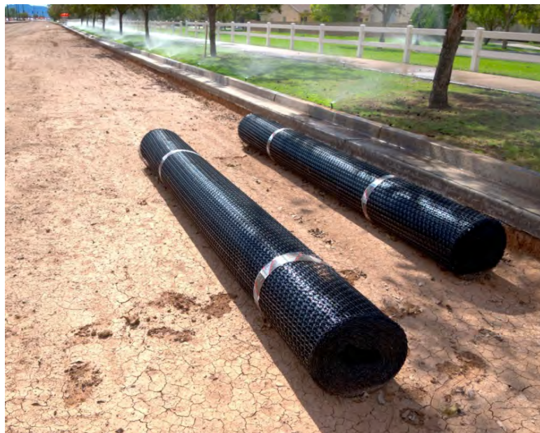
Photo No. 1 - Rolls of Geogrid
