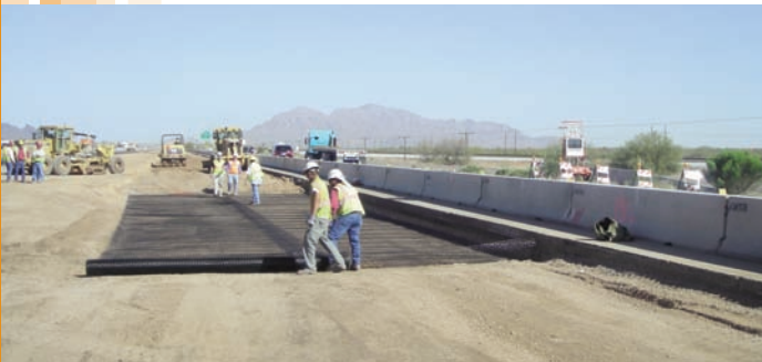
Tensar® TriAx™ Geogrid delivered an affordable option to remediate problem areas with weak soils.
