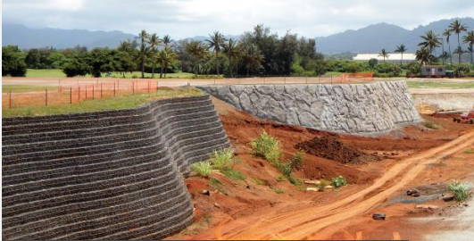
Geogrid reinforced retaining walls (stone-faced or vegetated face)
