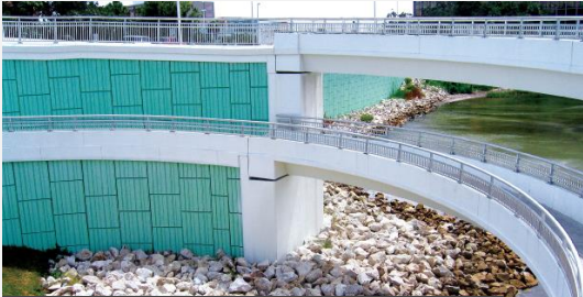
Geogrid reinforced precast panel system
