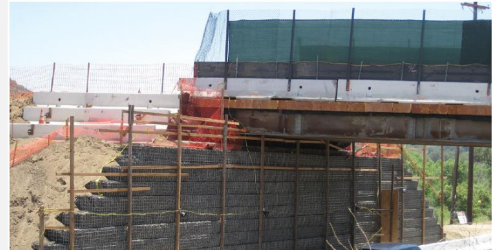
Tensor was able to create true abutments with the ability to handle very large surcharge loads.
