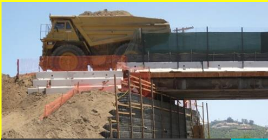
Temporary wall systems
