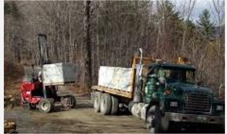
Typically about 500 blocks/truck 500 SF of wall face
