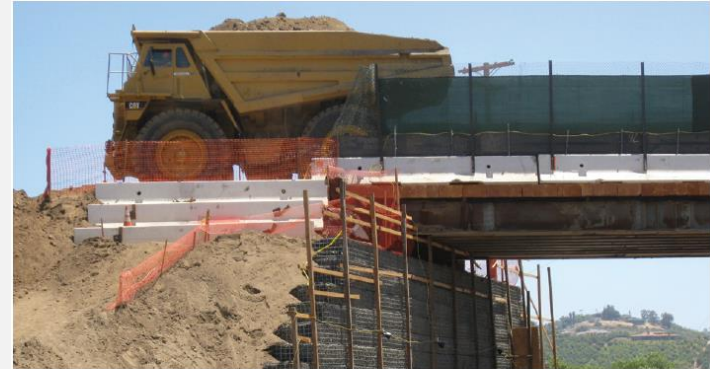
A CAT 777 weighing approximately 360,000 lbs is supported by a Tensor Temporary Wall as it drives to the embankment site.
