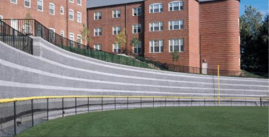
Segmented block retaining wall system
