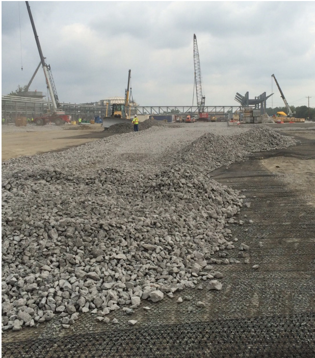
Base aggregate is installed over Tensar® Geogrid.
