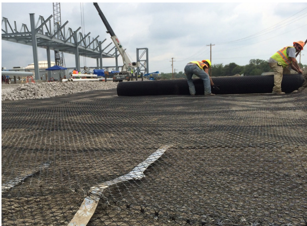
Workers begin the placement of the Tensor® TX5 Geogrid .
