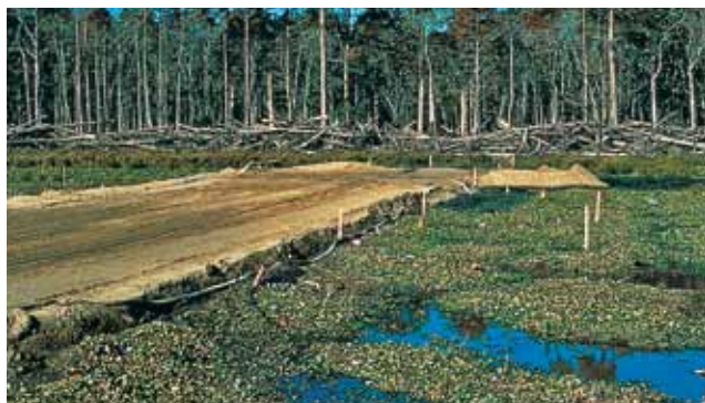
Dique de Westminster – Jefferson Parish, Louisiana
