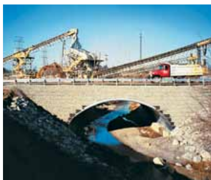
Vulcan Materials Plant – Columbia, Carolina do Sul
