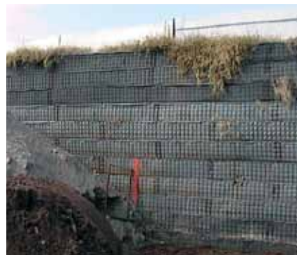
Ringling Causeway Project – Sarasota, Florida
