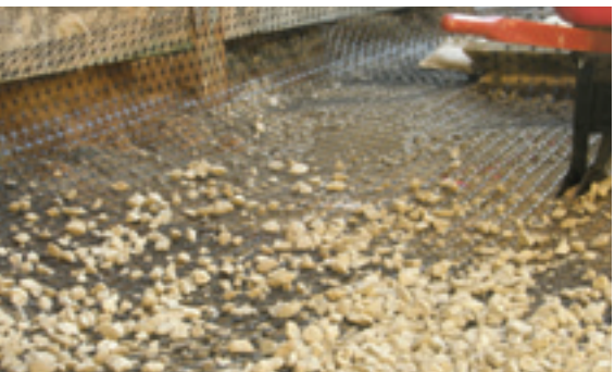
Los Angeles Museum of the Holocaust – Los Angeles, CA The Dimension System was used to create a foundation improvement solution for the facility. A Mechanically Stabilized Earth (MSE) mattress offered an affordable alternative to overexcavation and replacement while also minimizing differential settlement.
