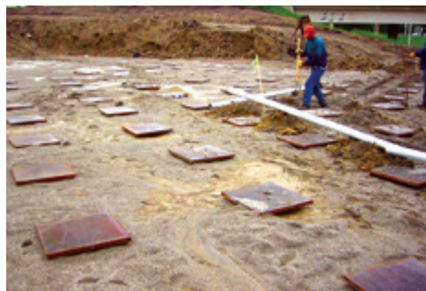
This photo and diagram are examples of an LTP System and soil arching.
