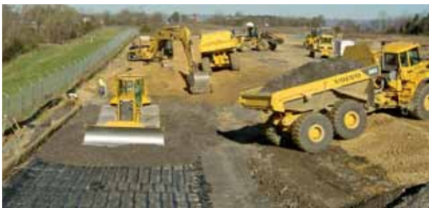
Standard construction techniques with proven MSE technology.
