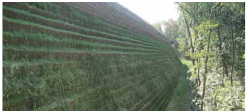
ADD 3 steep berms increase landfill capacity within boundary constraints.
