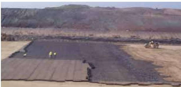
Tensor UX Geogrids can protect the integrity of lining systems by managing lateral strains created by new landfill construction.
