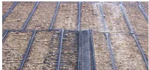
Tensor UX Geogrid structural connections minimize waste factors.
