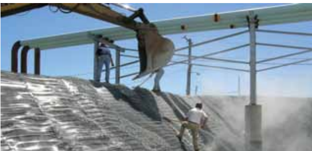
Their pronounced and more closely spaced transverse bars makes the Tensar SB products ideal for veneer stability applications.
