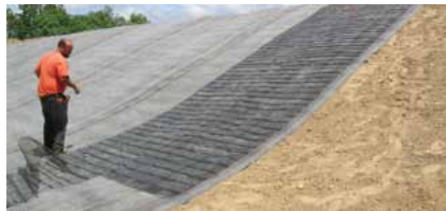
Their pronounced and more closely spaced transverse bars makes the Tensar SB products ideal for veneer stability applications.
