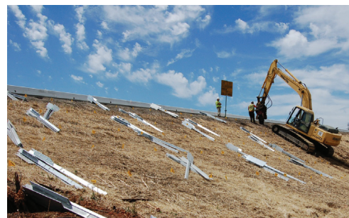
Williams, California: Stabilizing 1.5 miles of embankment slopes for Caltrans using Geopier® Plate Piles™.
