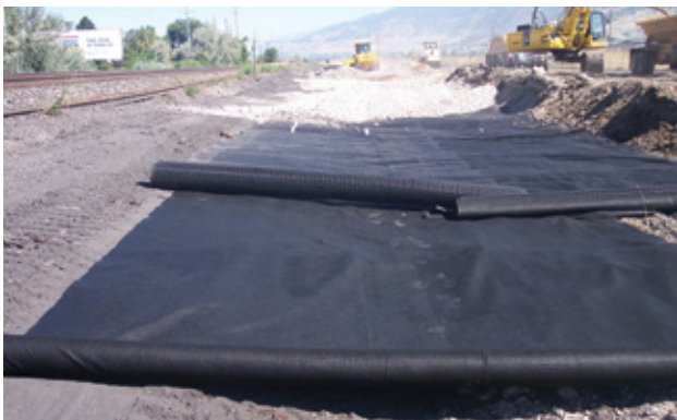
The transition zone is stabilized by incorporating Tensar's Geogrid.
