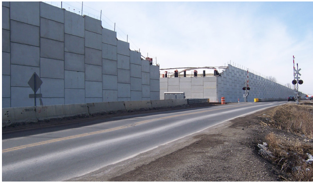
ARES Systems, utilizing Tensar Uniaxial Geogird reinforcement, can be used in a wide variety of backfill materials, including pH extremes, sulfates and where resistivity is an issue. This advantage allows for use of locally available materials to save on construction costs.
