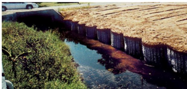
*Triton Circular Marine Cells anchored by Tensar® Geogrid, provide economical, easy-to-install solutions for applications like this channel wall in a residential community.*
