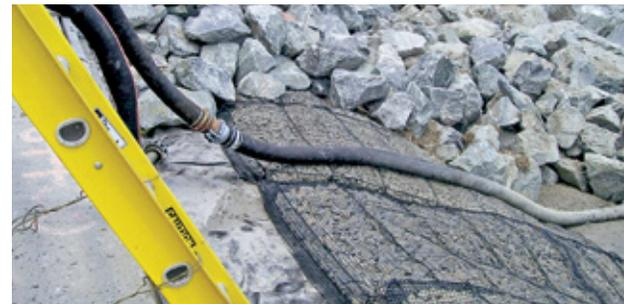
*As a revetment foundation, the Filter Mat provides bedding and filtration, helping to prevent differential settlement. The mats also protect against scour at the toe of the revetment.*
