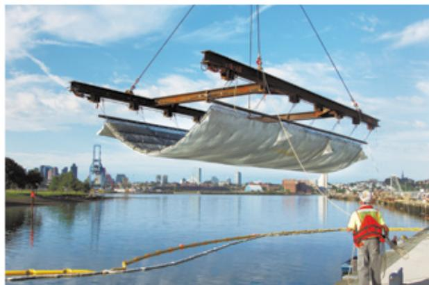
*Triton Marine Mattresses have been used to provide effective capping for a wide range of contaminated sediment projects.*
