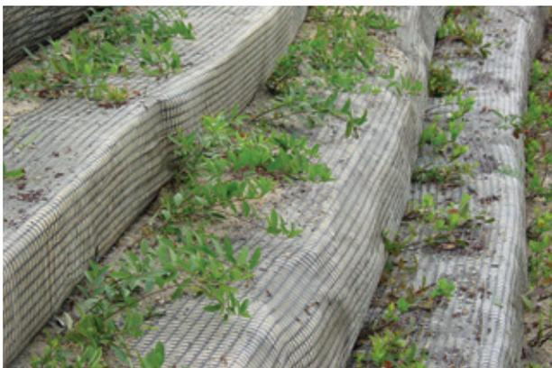
Tensar® VRSS promote the propagation of native vegetative root systems to strengthen reinforcement structures over time.
