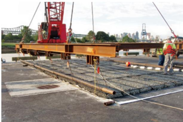
*Triton® Marine Mattresses have been deployed as part of a reactive capping system for the remediation of NAPL when used with CETCO® Reactive Core Mats.®*
