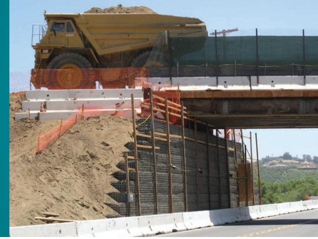
The photo to the left illustrates a CAT 777 weighing approximately 360,000 lbs that is supported by a Tensar Temporary Wall as it drives to the embankment site.
