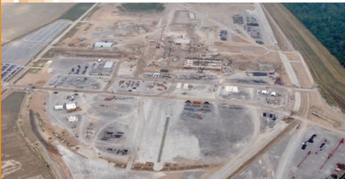
Plum Point's cotton fields are transformed into high capacity working surfaces by Tensar Geogrids, sand subbase and crushed limestone base.
