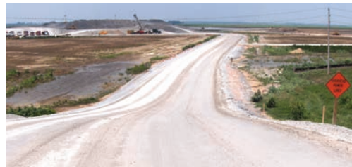
Main haul/access road held up well to high volumes of articulated truck traffic.
