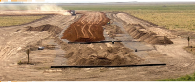
Main haul/access road with two layers of Tensar Geogrid sandwiching sand subbase and topped with crushed limestone base.
