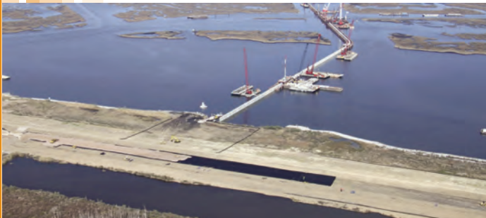
The principle working surface of LPV-145 shown above. Here, geogrid is atop geotextile with sand subbase being advanced over the geosynthetics from left to right.
