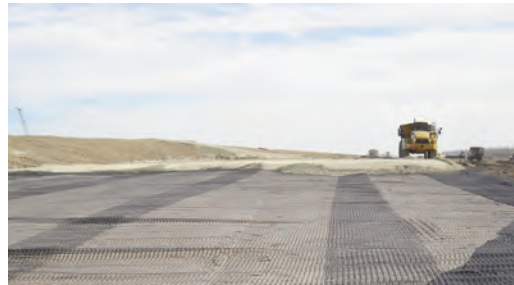
Locally dredged river sand was sandwiched between two layers of Tensar Geogrid (upper layer shown) and topped with crushed granular fill (in background).
