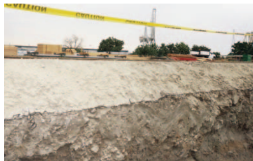
Excavation revealed the nominal 12-in.-thick section of imported crushed aggregate atop Tensar BX1200 Geogrid. Geogrid reinforces the aggregate and separates it from the underlying cohesive soils.
