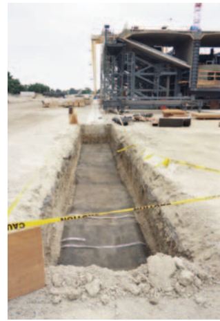
A gantry crane foundation was extended part-way into the project.
