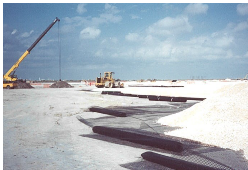
Installation of Tensar Geogrid at the site of Kiewit Offshore Services in 2001.
