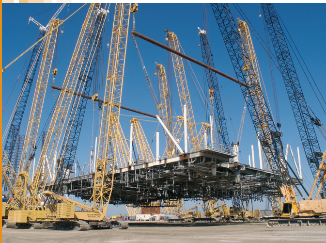
Working surfaces have held up well to heavy, live loads.
