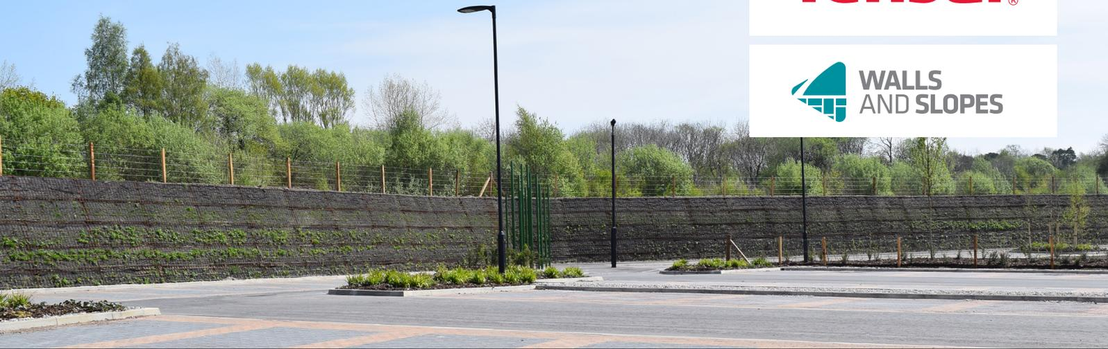
Tensar's TensarTech GreenSlope system was used to build the 70° slope, maximising car parking space, with a natural, vegetated finish helping it to blend into the surrounding landscape.
