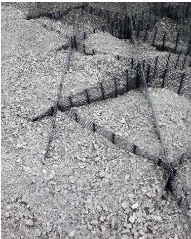
The cellular structure of TensarTech Stratum under construction
