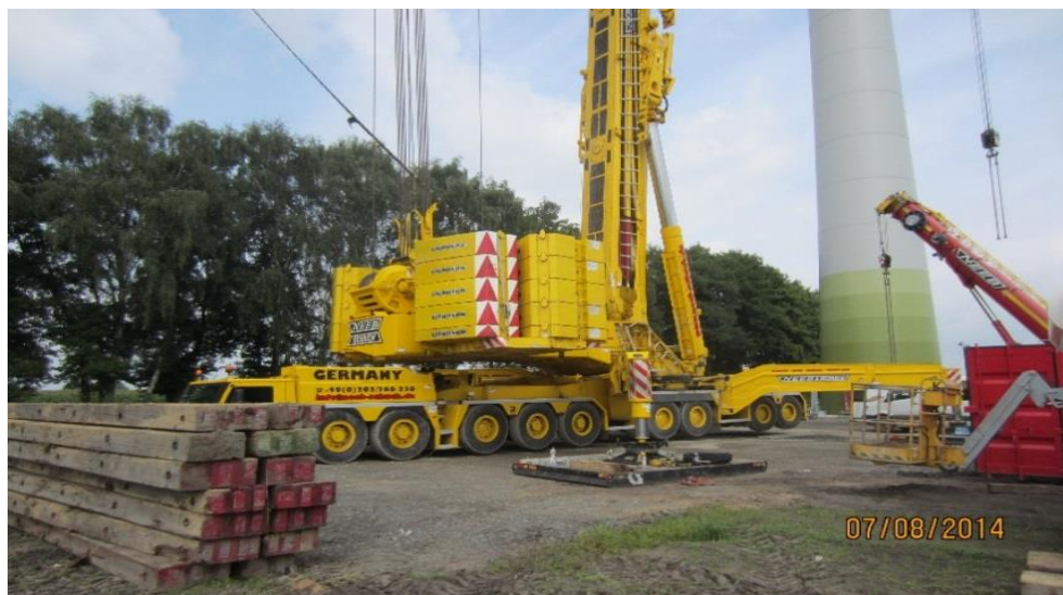
Heavy lift crane operating on completed TensarTech Stratum working platform
