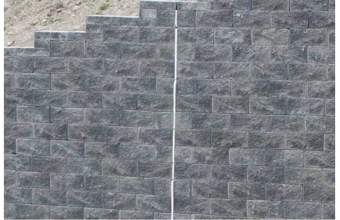
Figure 13. Slip joint pre-earthquake
