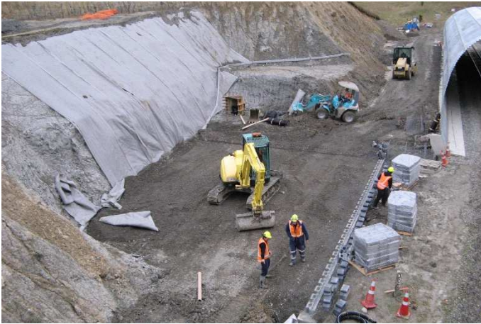
Figure 5. Modular block east wall at Dashwood at early stage
