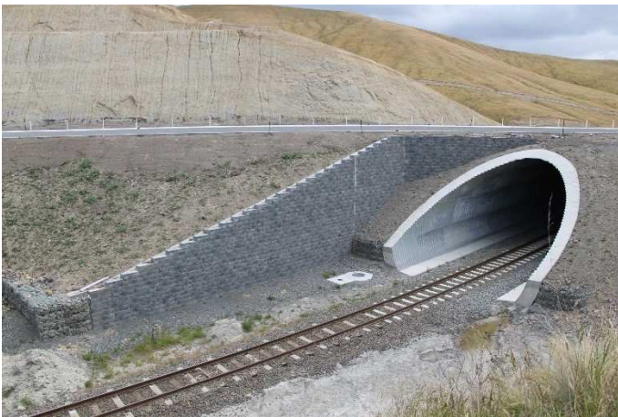
Figure 6. Modular block west wall at Dashwood completed
