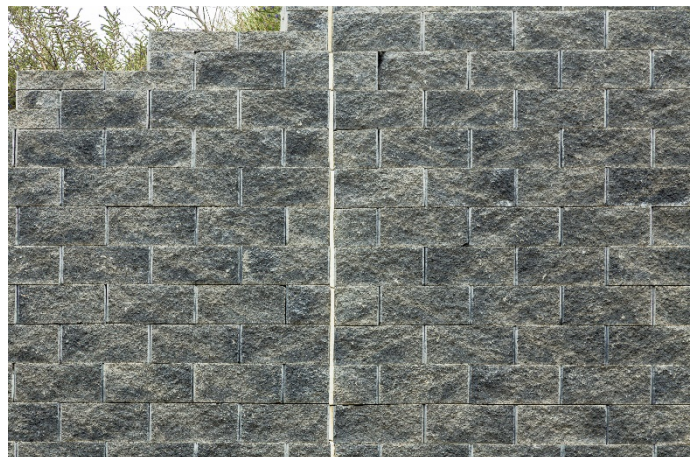
Figure 14. Slip joint post-earthquake
