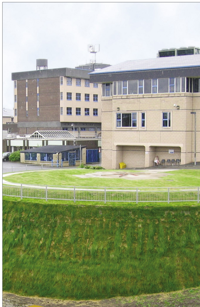
Tensartech GreenSlope technology created this helicopter ambulance landing site.
