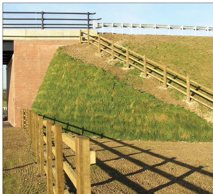
This geogrid stabilised slope is part of a road bridge abutment.
