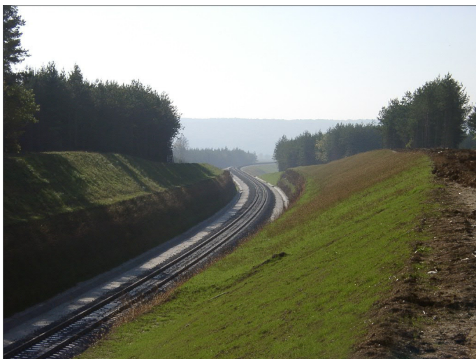
TensarTech GreenSlope reinforced soil system stabilising a steep roadside structure.
