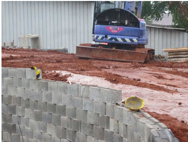
Figure 21: Bridge approach structure built in Tangerang using tanah merah backfill
