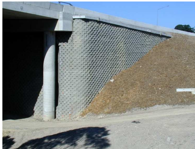
Figure 14: Bridge abutment in New Zealand built using weathered Waitemata Clay residual soil
