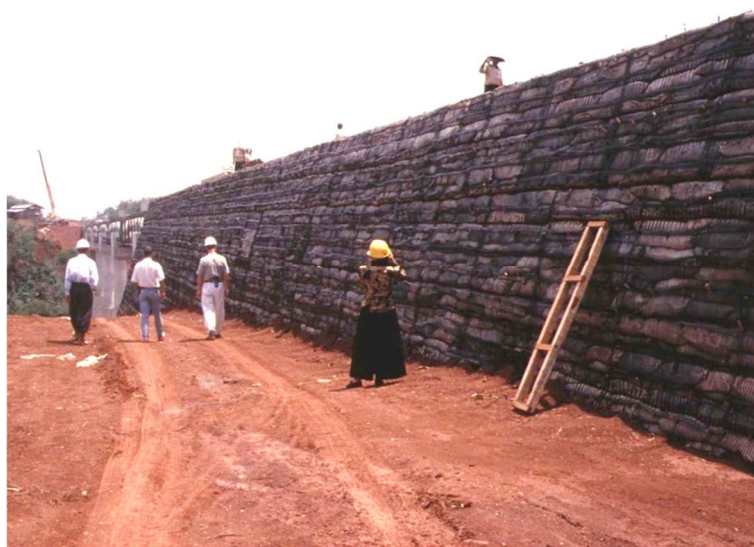
Figure 19: Reinforced soil steep slope carrying railway loading built using tanah merah
