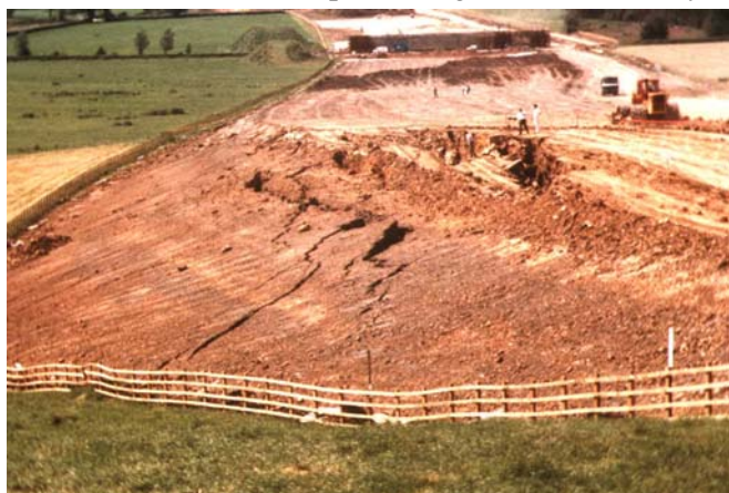
Plate 1 Failure of the Hill Hall embankment
